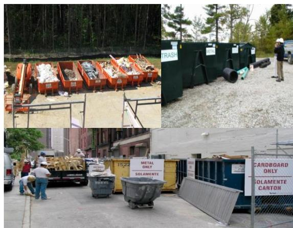
**Figure 4.** Initial separation of construction waste
