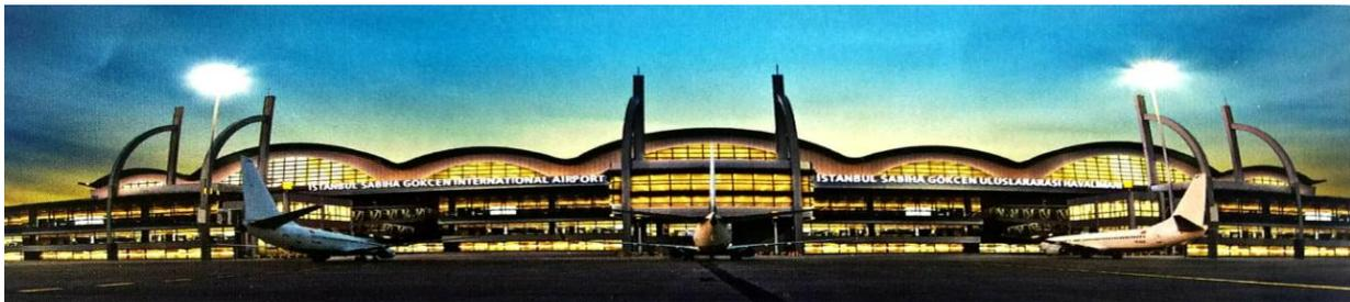
Picture 2 - Istanbul's Sabiha Gokcen international Airport Terminal, Turkey, one of the largest seismically isolated buildings in the world. Source: H. Darama, Arup
