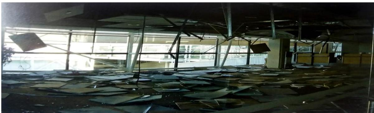
Picture 3 - Non-structural damage to a suspended ceiling at the Santiago International Airport terminal building after the 27 February 2010 Chile earthquake. Source: G. Mosqueda
