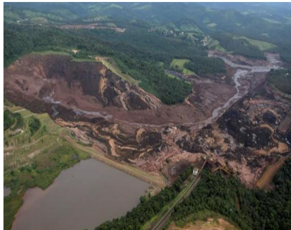
d) The dam was 87 m high, impounding almost 13 million cubic meters of tailings.
