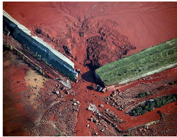
b) Kolontar tailings dam failure in Hungary, 2010
