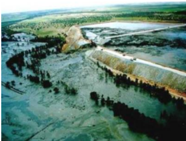
a) Los Frailes mine tailings dam in Aznalcóllar, Spain, 1998
