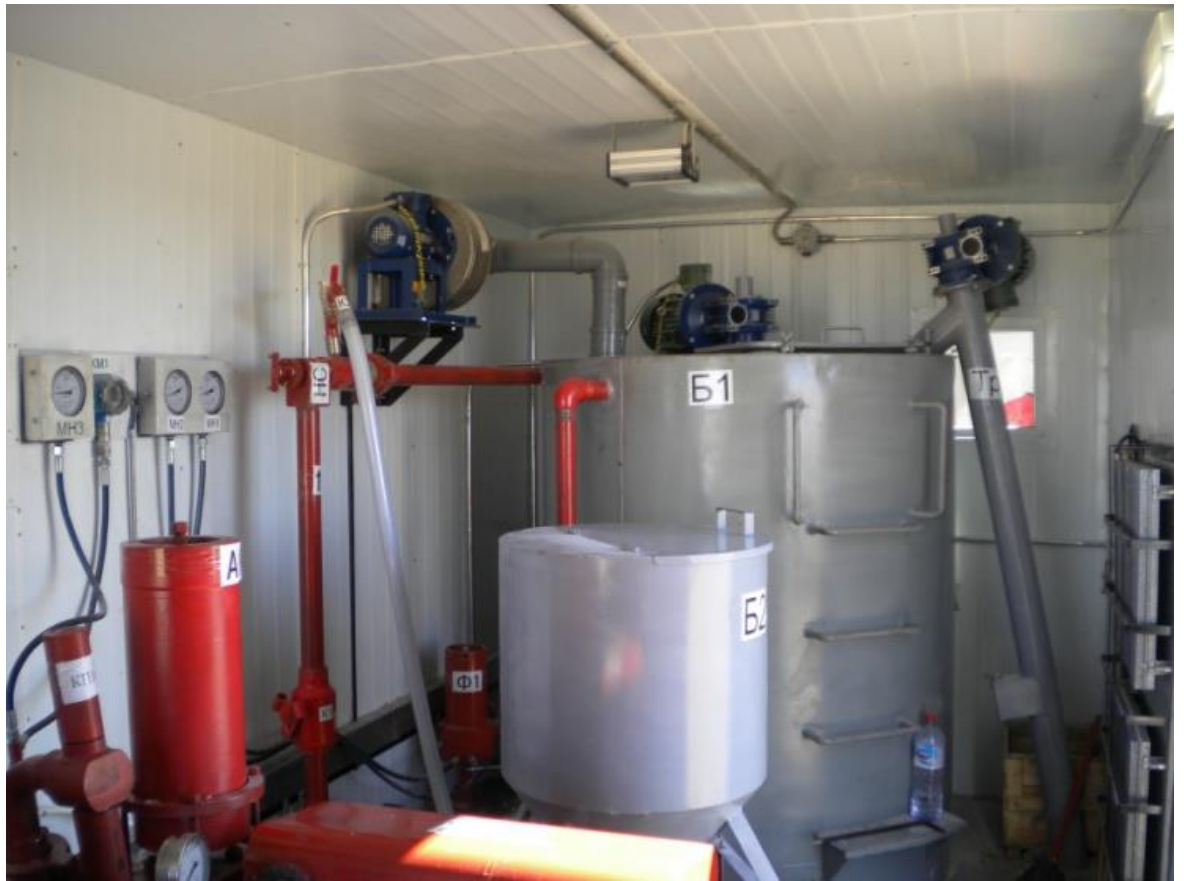
Figure 53 - КУДР - complex equipment for dosage of chemicals.
